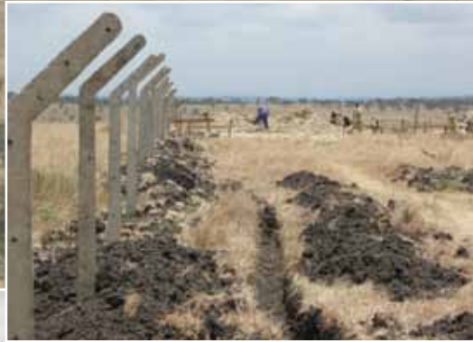
A security fence marks the perimeter of the Shunem property.
